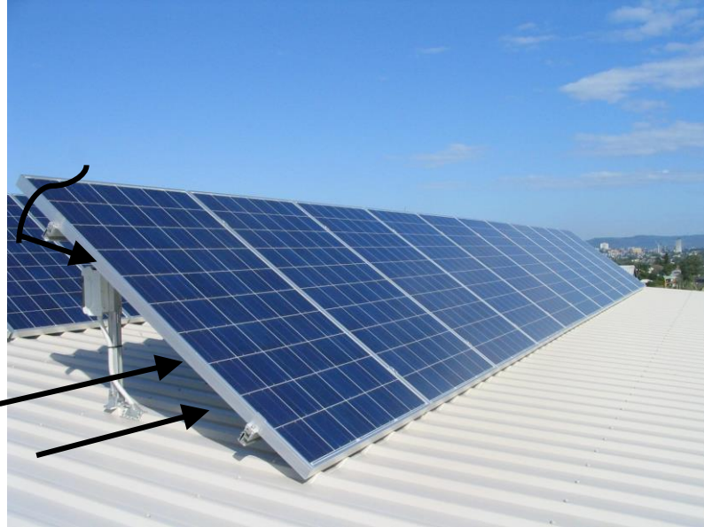
Total load on Roof = Static Load + Dynamic Wind Load
